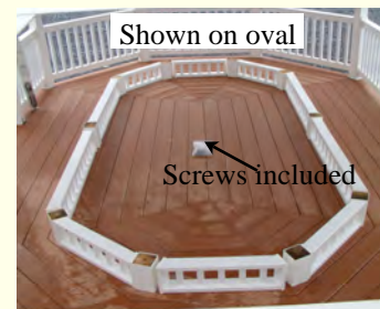
D=laying out the short spindles before installing
