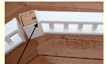
C=Short spindle with electrical wiring channel
